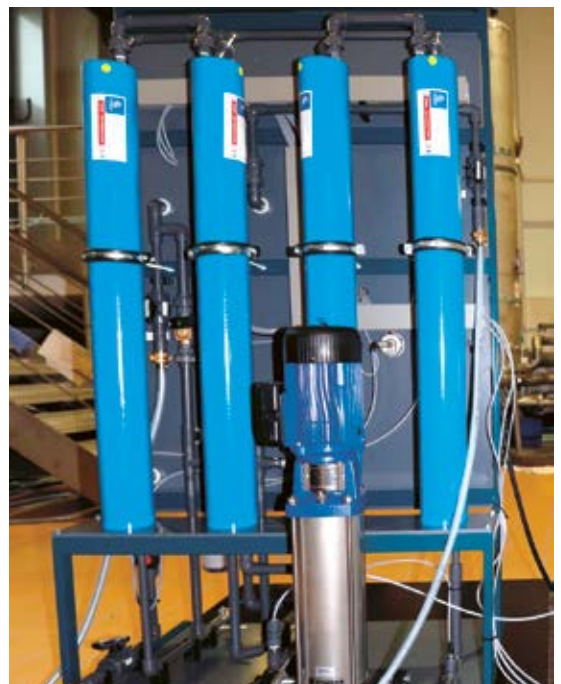
Pilot plant of low-pressure reverse osmosis at water works Berlin-Friedrichshagen (front and back view)
