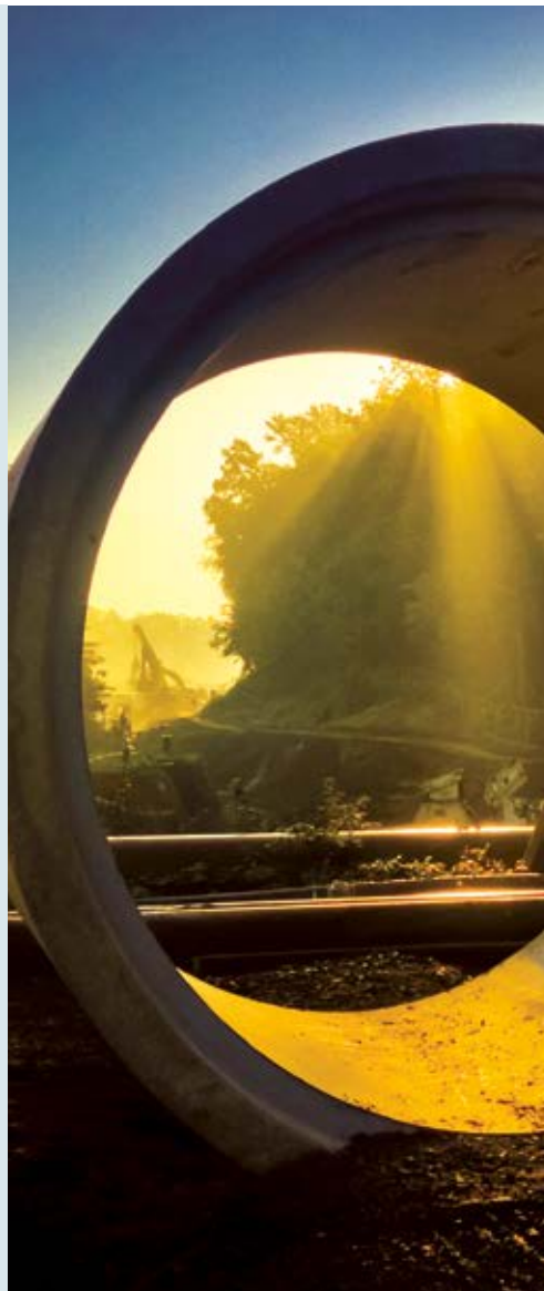
Installation of a sewer network
