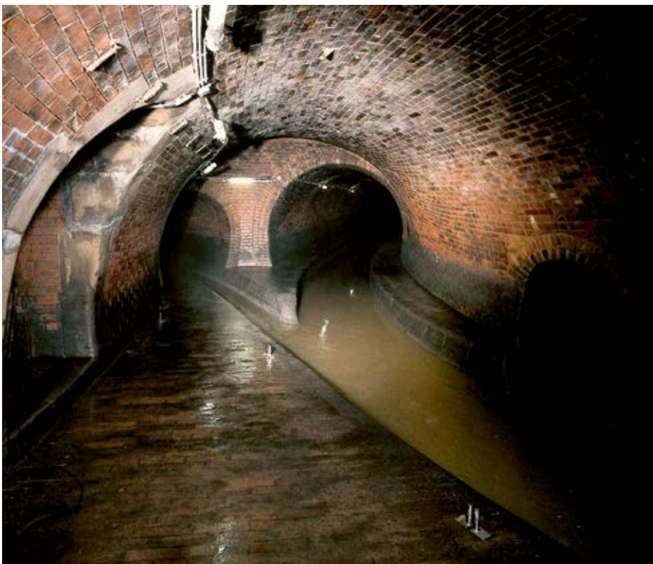
View to a combined sewer system in Berlin
