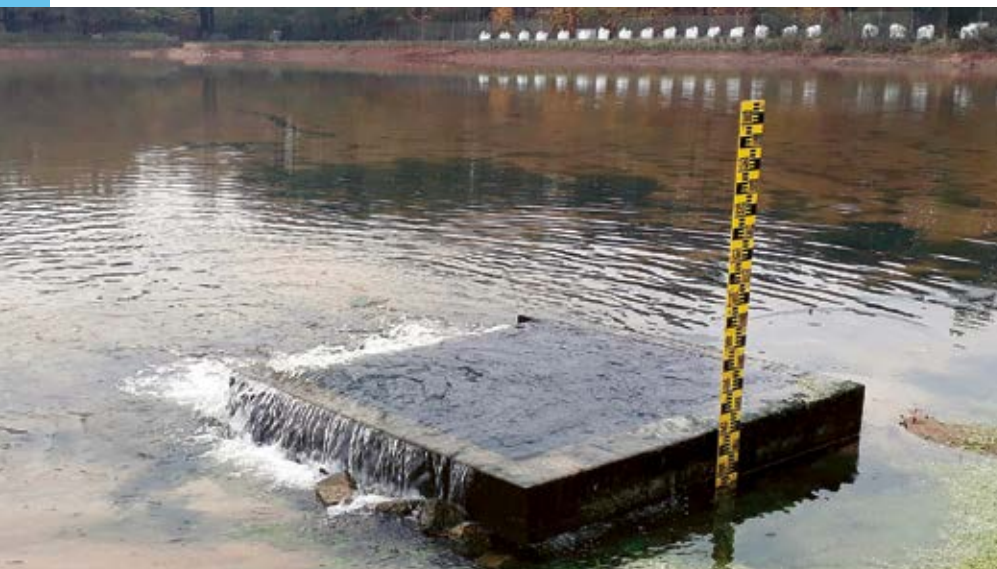
Groundwater augmentation pond at waterworks Berlin-Spandau
