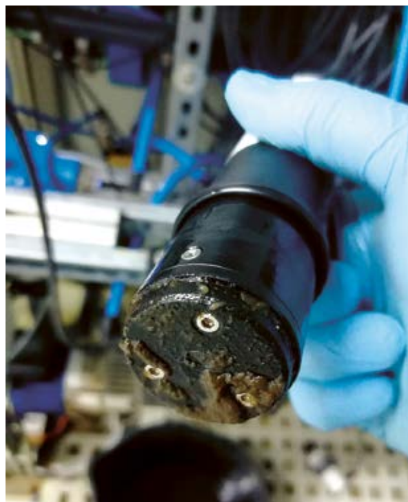
Online sensor installation in a pilot ozone system at WWTP Schönerlinde
