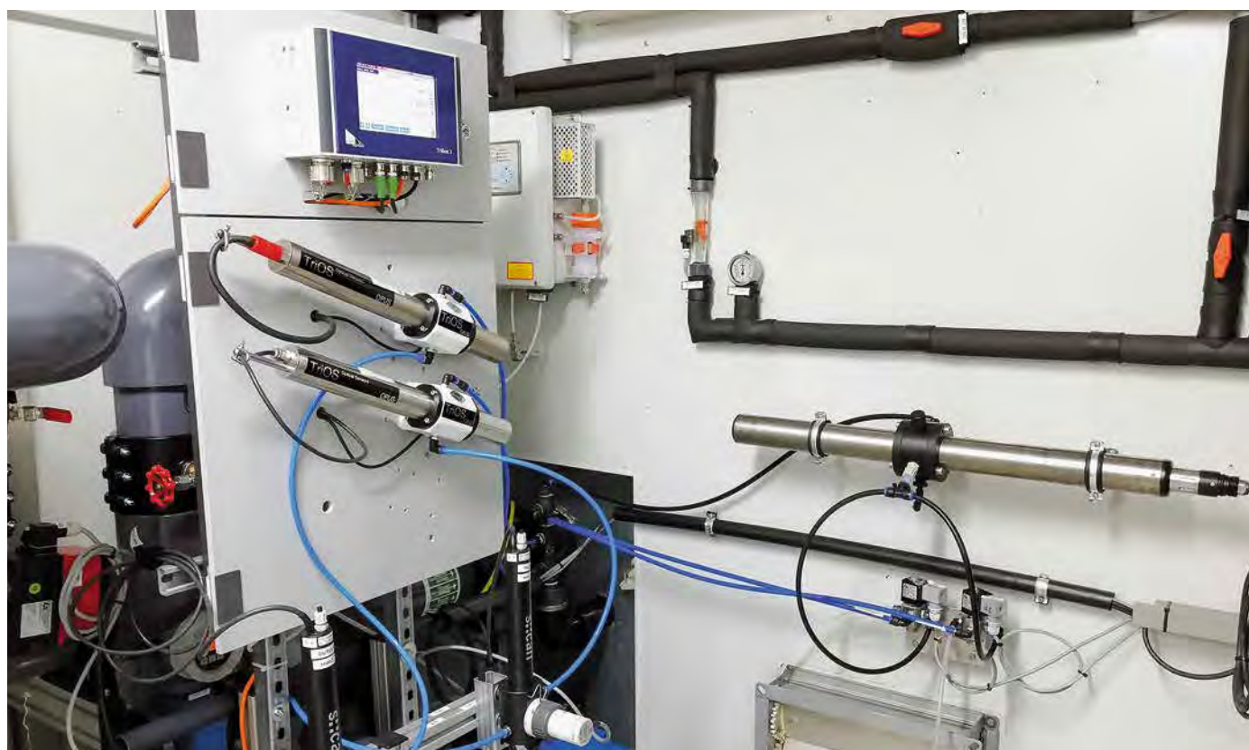
UV-VIS-Sensors installed in the ozone pilot plant
