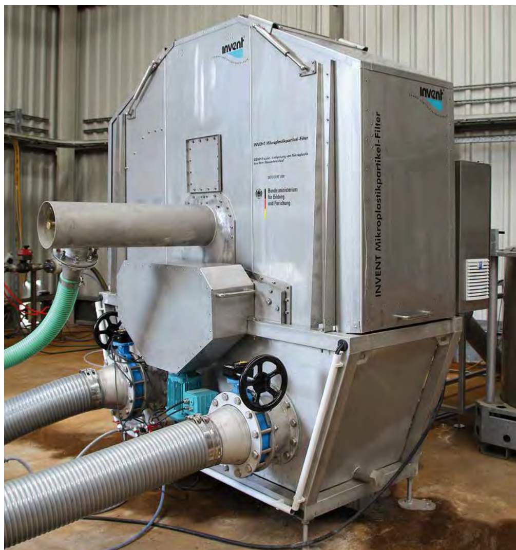
Pile cloth media filtration pilot unit at WWTP Ruhleben, Berlin
