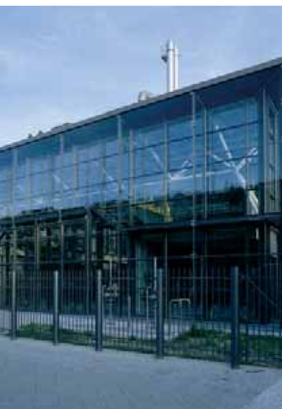
Abwasserpumpwerk Sewage pump station
