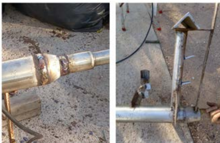
Figure 12 Reinforcement of mixing arm by double welding in two positions
