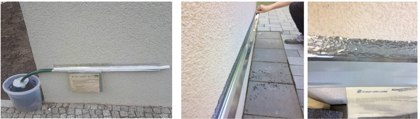
Figure A2. Installation of a gutter to capture façade runoff.
