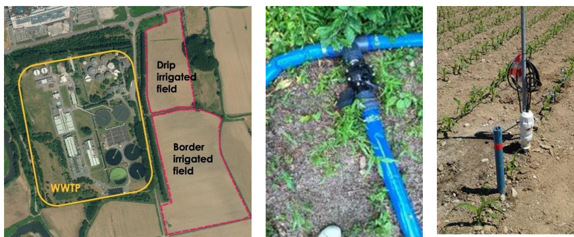
Figure 40: Overview of demo site (left), drip irrigation system installation (center), piezometer, water content probe + GSM modem, porous cups (right).
