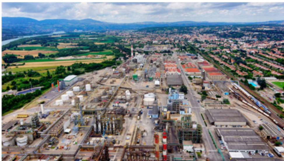
Figure 103. The Roches-Roussillon chemical platform.
