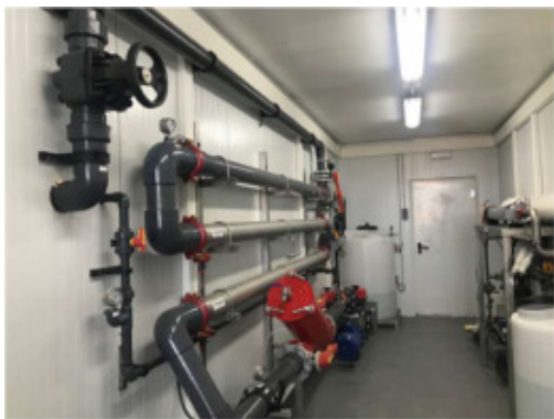
(c) Ultrafiltration process
