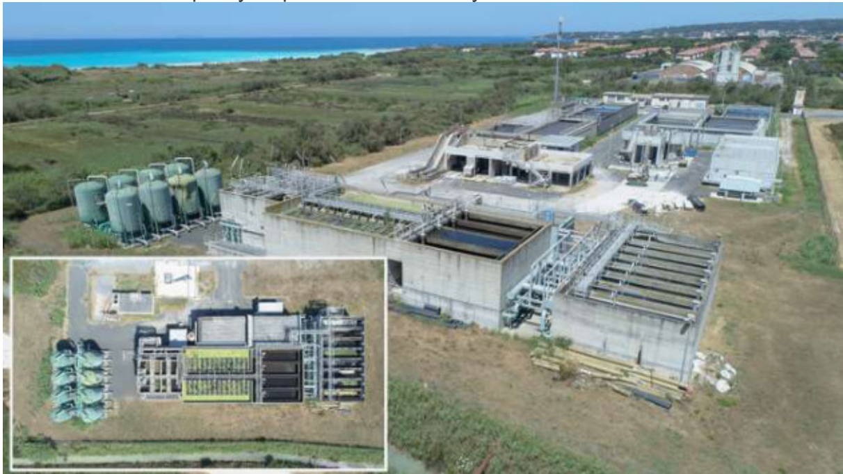
Figure 30. ARETUSA WRP in Rosignano WWTP Area.
