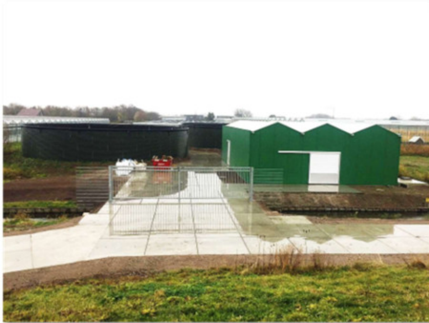
Figure 20. Treatment plant De Vlot.
