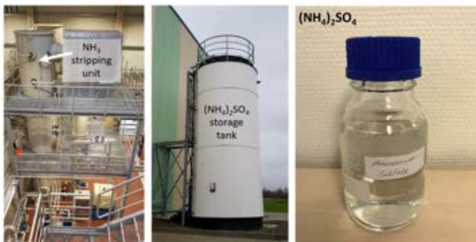
Figure 42 Pictures of the ammonium sulphate production units, the storage tank and an ammonium sulphate solution sample
