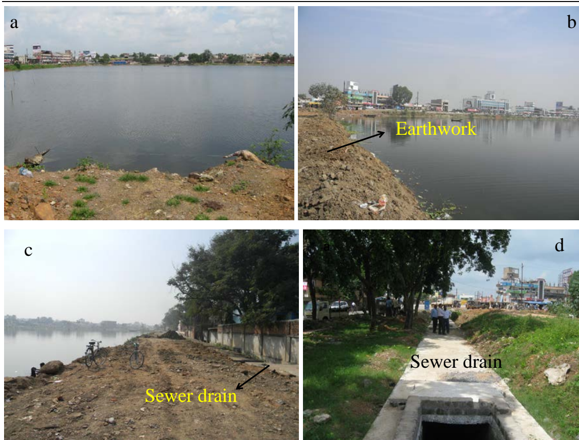
Figure 29 Photographs show views of the Teliabanda Lake and its on-going rejuvenation works: (a) a view of the lake during monsoon season (August, 2012) (b) showing earthwork along the lake boundary; (c) a view of the earthen embankment and diverted sewer drain; and (d) a view of the diverted sewer drain.
