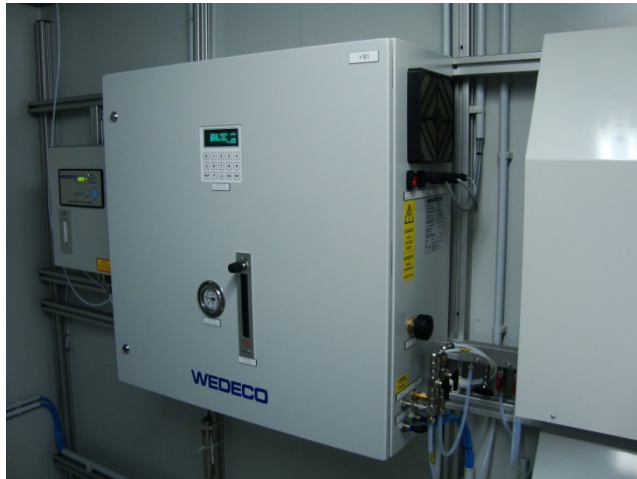
Figure 6: Ozone generator and bubble column
