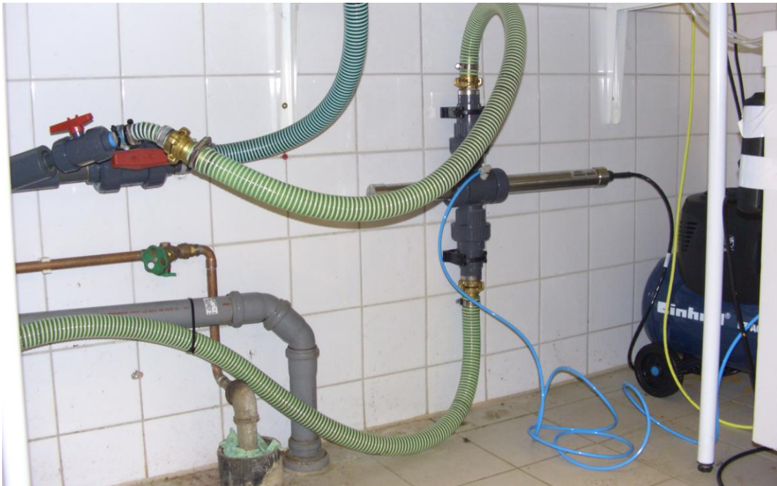
Figure 16. Location and probe's installation at the upstream river monitoring station 1
