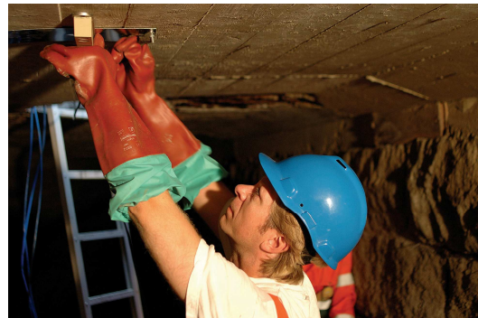
Installation of ultrasonic sensor
