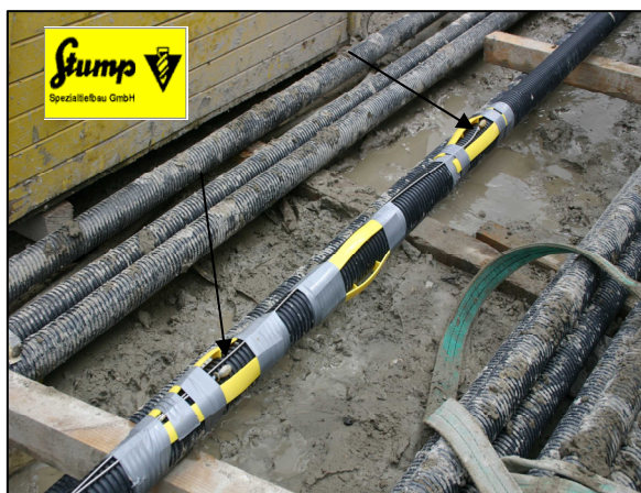
Figure 12: Water filled topcoat for the pH-sensitive membrane to prevent dehydration. Photo: STUMP GmbH
