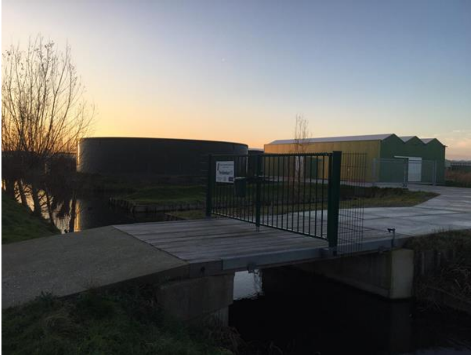
Fig. 5 De Vlot wastewater treatment plant facility
