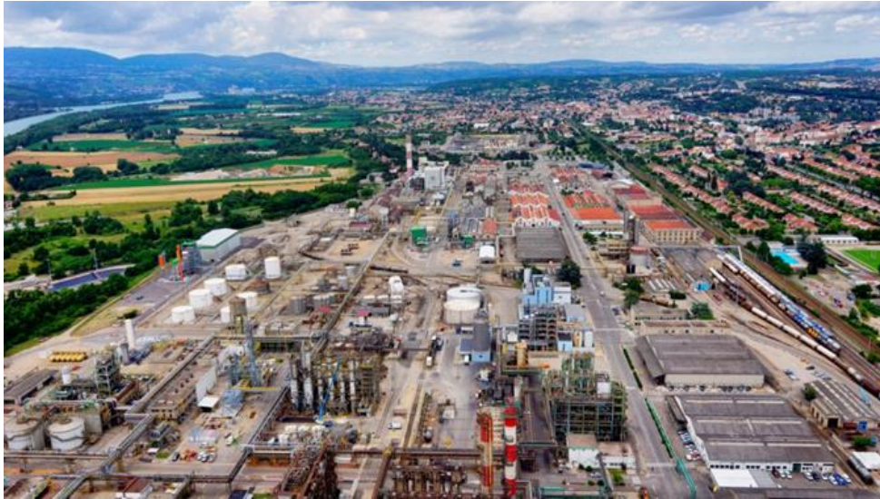
Fig. 16 The Roches-Roussillon chemical platform
