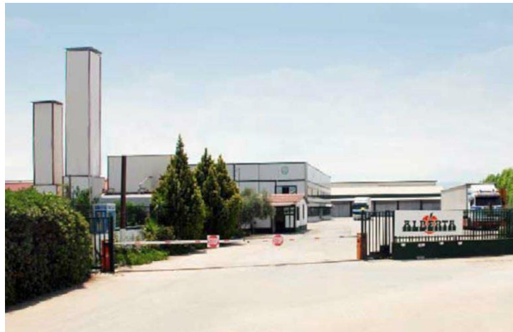
Fig. 10 Alberta S.A. facilities
