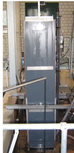
Figure 47. Installation of the A3 triple deck module in the pilot plant of Seelscheid WWTP
