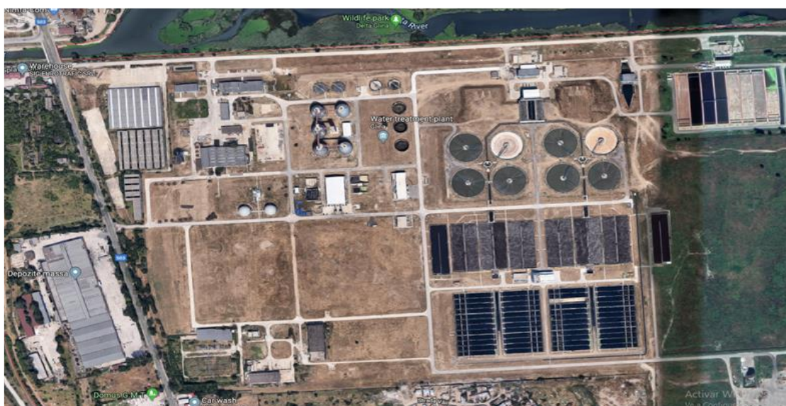
Figure 7. Aerial view of the Glina WWTP (source: google maps).
