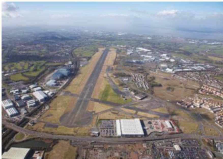
Figure 13. Aerial view of the Filton Airfield.
