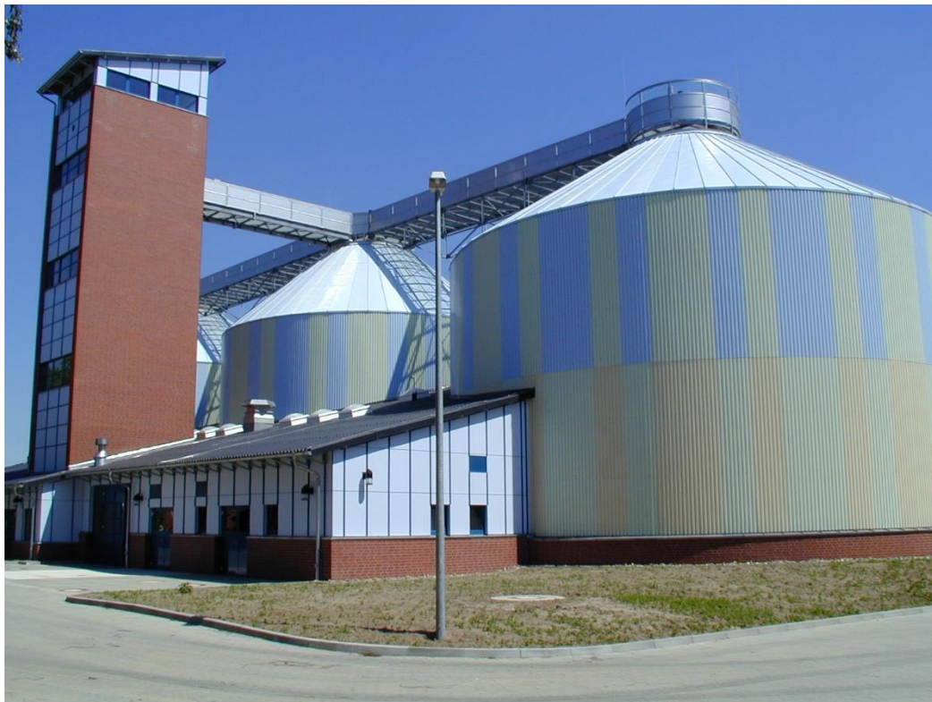
Figure 5. Picture of the three digesters at the WWTP in Steinhof near Braunschweig.
