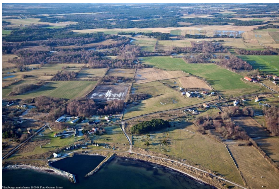
Figure 17. Picture of the site.
