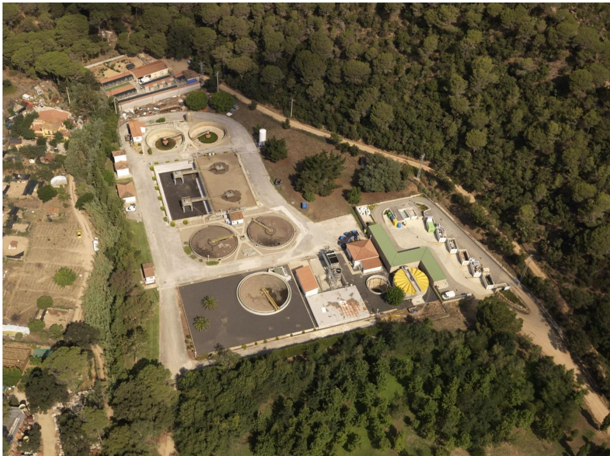
Figure 10. Aerial view of the WWTP of Tossa de Mar.
