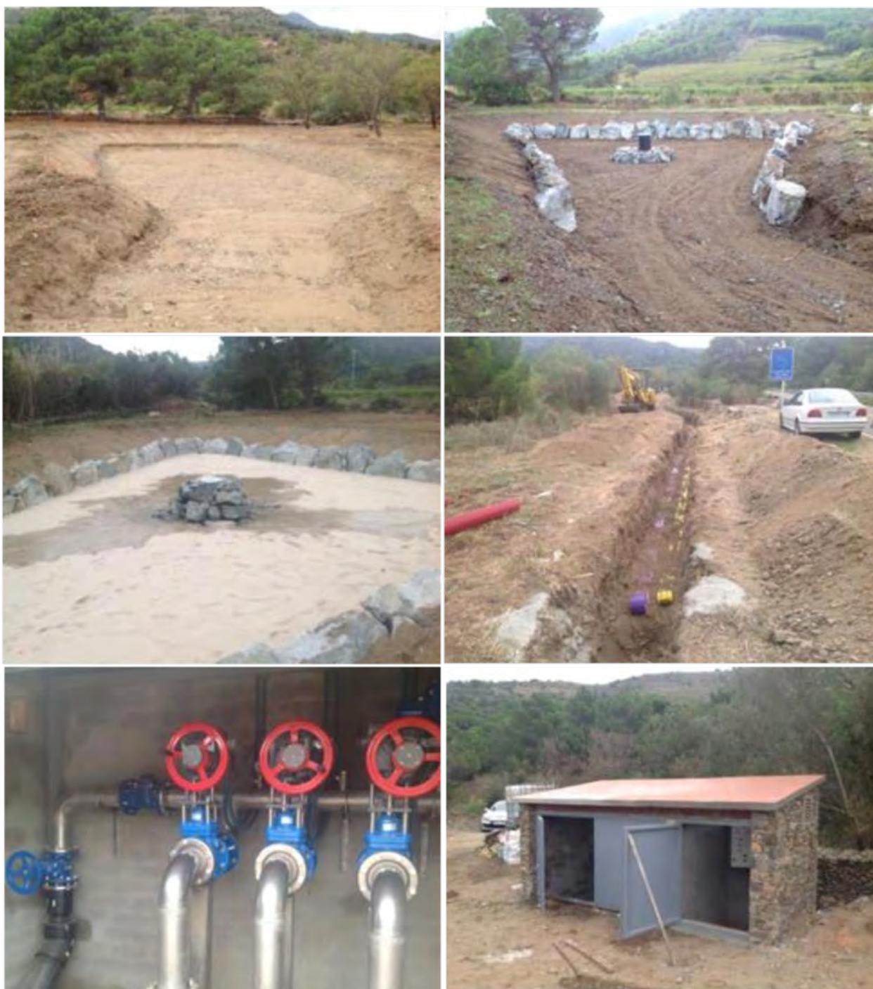
Figure 36 Work in progress.
