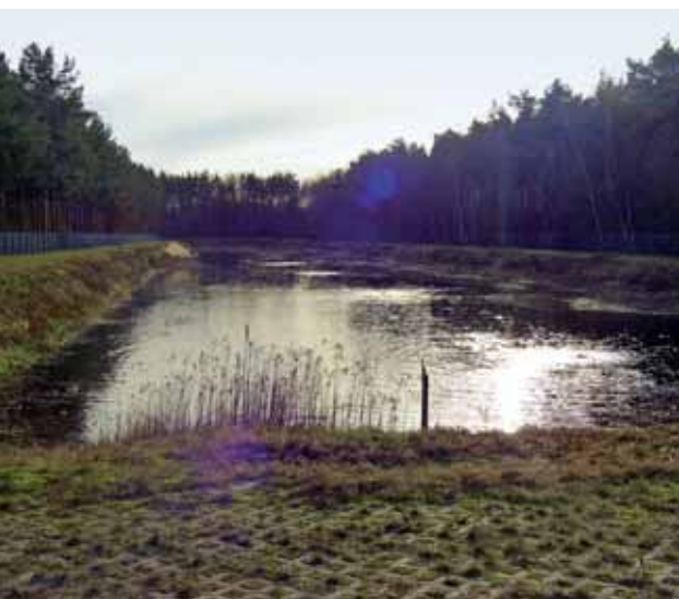
Picture 1 Artificial recharge pond at Spandau waterworks (Berlin)
