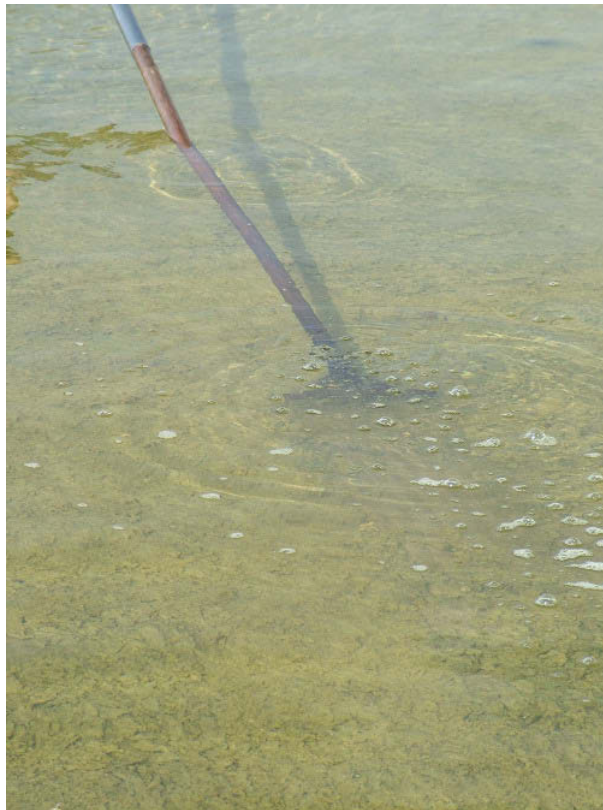
Figure 40: Photograph taken during raking of the SSF in order to destroy the superficial clogging layer.
